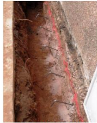
P4 – Dowel bars into existing foundations
