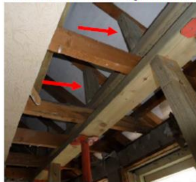
P6 – First floor propping with vertical support to roof rafter:
