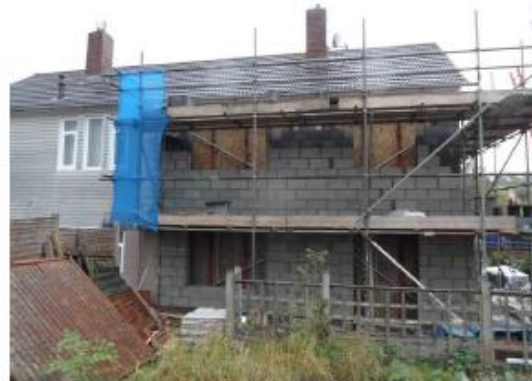
P12 – External Walls
